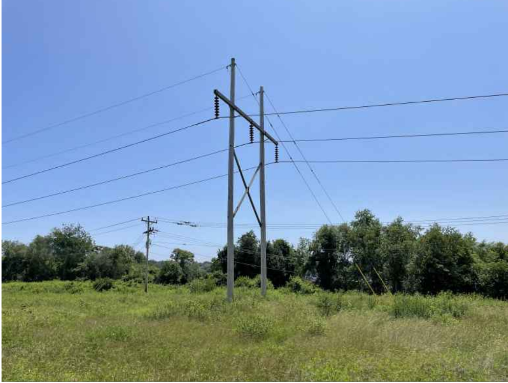
Photograph No. 27: Looking south at Structure 5 on the T13 Line ROW off Gosling Road, Portsmouth, NH.
