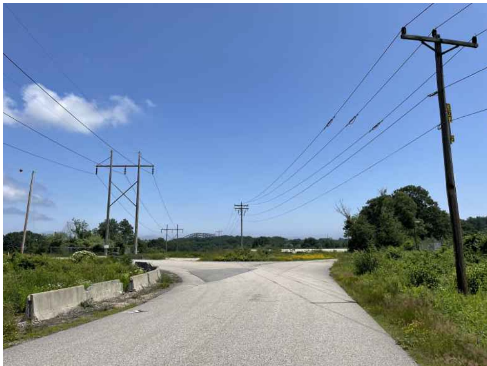
Photograph No. 30: Looking east at Structure 7 and Wetlands PW-10 (PSS1Ex) and PW-11 (PSS1/PEM1Ex) on the T13 Line ROW off Gosling Road, Portsmouth, NH.
