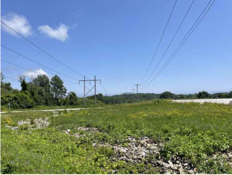
Photograph No. 31: Looking east at Wetland PW-11 (PSS1/PEM1Ex) between Structures 7 and 8 on the T13 Line ROW off Gosling Road, Portsmouth, NH
