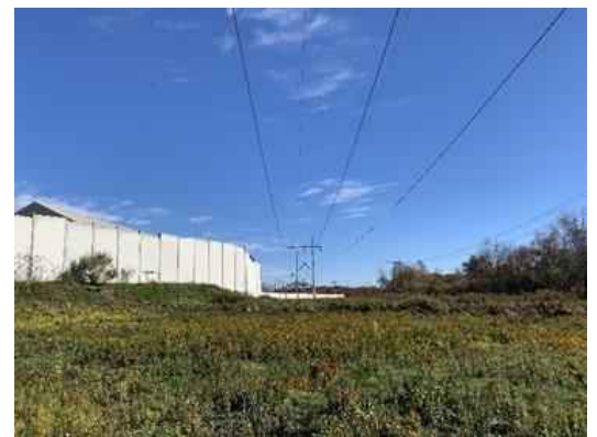
View of ROW facing east toward T13 Structure 6.
