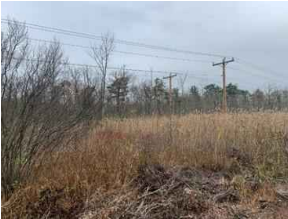
View of ROW facing north toward Line 3171 Structure 82.
