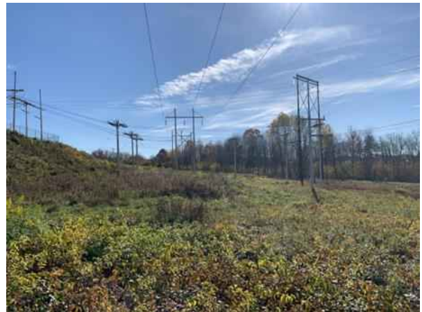
View of ROW facing south toward line T13 Structure 3.
