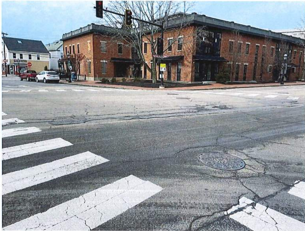
Photo 19 – Maplewood Ave and Hanover Street intersection looking south. Taken 1/19/23
