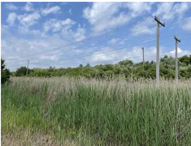
Existing wooden Structure 81 on 3171 Distribution Line.
