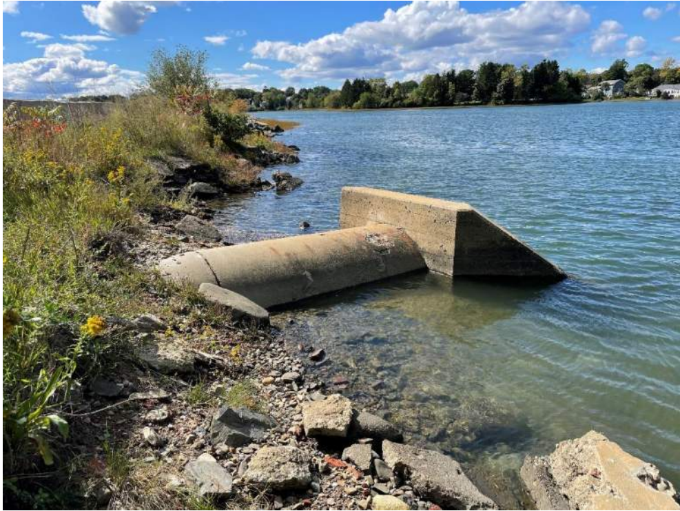
Photo 1 – Existing outfall headwall, exposed 48” RCP pipe, and tidal embankment looking west at approximate high tide. Taken 9/28/22
