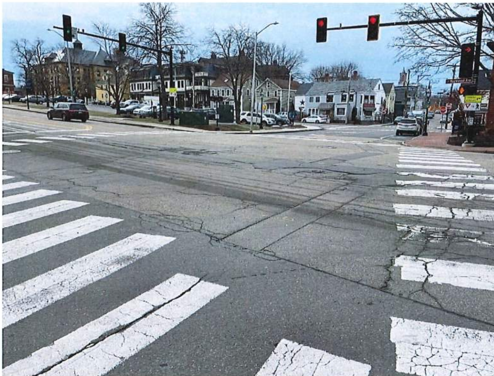
Photo 18 – Maplewood Ave and Hanover Street intersection looking east. Taken 1/19/23
