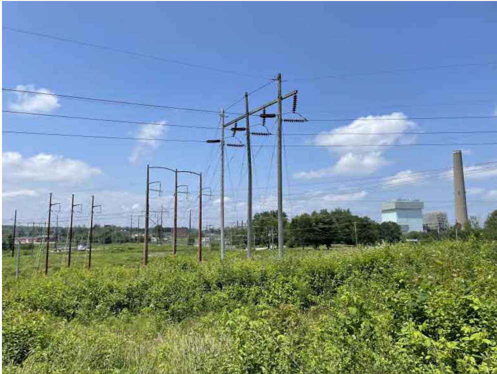
Photograph No. 21: Looking northwest near Wetland PW-3 (PEM1/PSS1E) between Structures 1 and 2 on the T13 Line ROW off Gosling Road, Portsmouth, NH.
