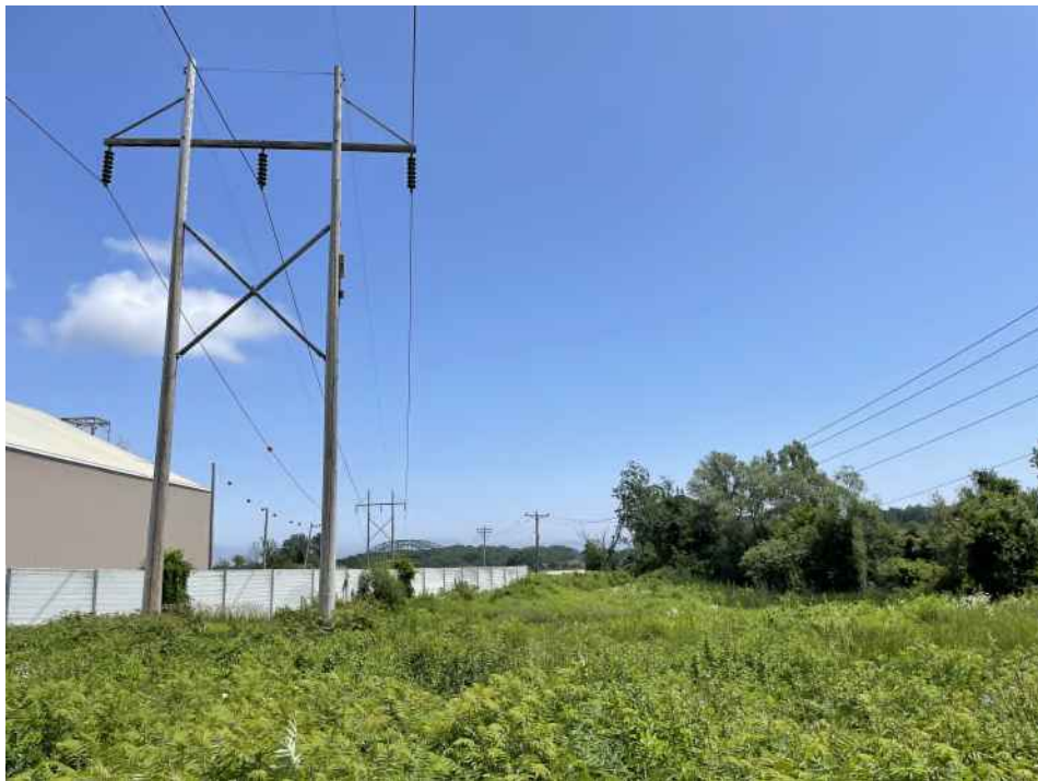
Photograph No. 28: Looking east at Structure 6 and Wetland PW-7 (PEM1/PSS1E,H) on the T13 Line ROW off Gosling Road, Portsmouth, NH.
