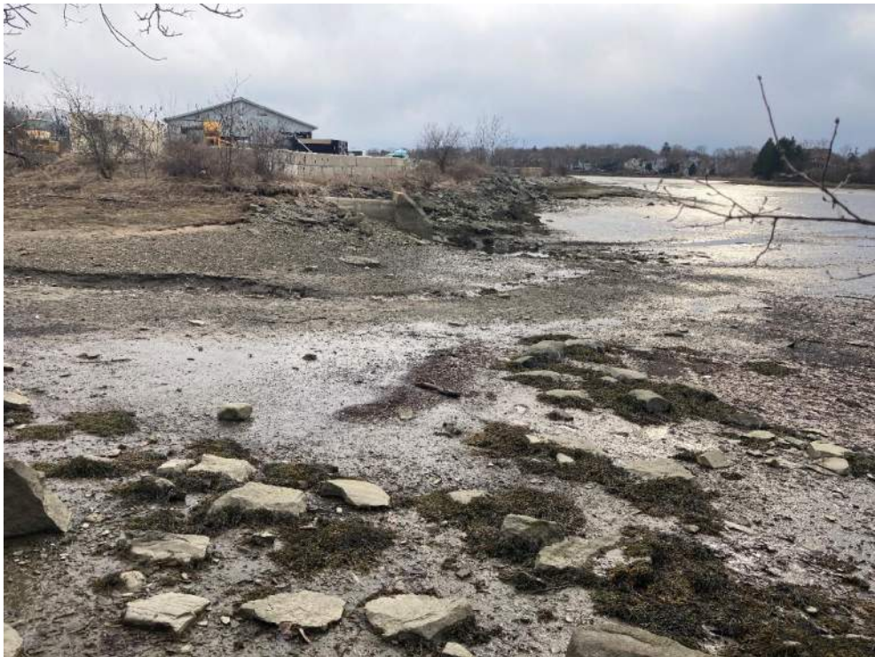
Photo 8 – Mitigation area, looking southeast at approximate low tide. Note existing large rocks to be stockpiled for use on stabilized slope and ice breakers. Taken 3/20/24
