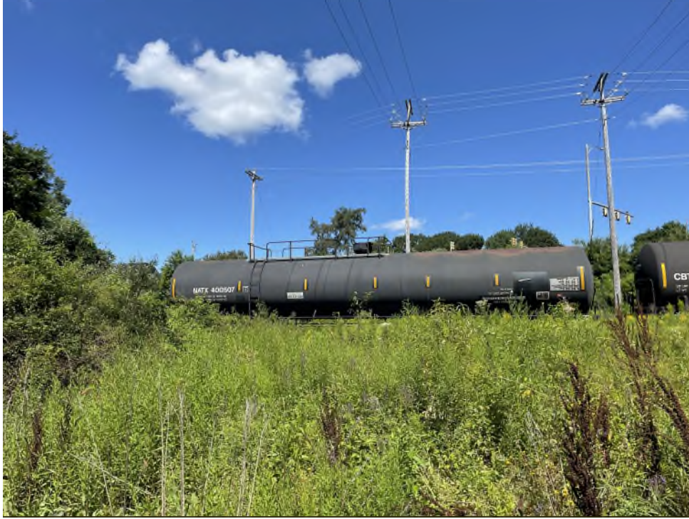
Photograph No. 17: Looking northwest towards Structures 72 and 72.6 on the 3171 Line ROW off NH33, Portsmouth, NH.
