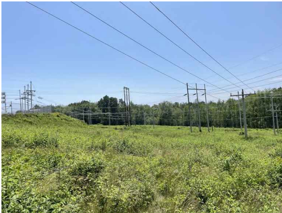
Photograph No. 24: Looking south at Structure 3 and Wetlands PW-5 (PEM1/PSS1E) and PW-6 (PEM1/PSS1E) on the T13 Line ROW off Gosling Road, Portsmouth, NH.
