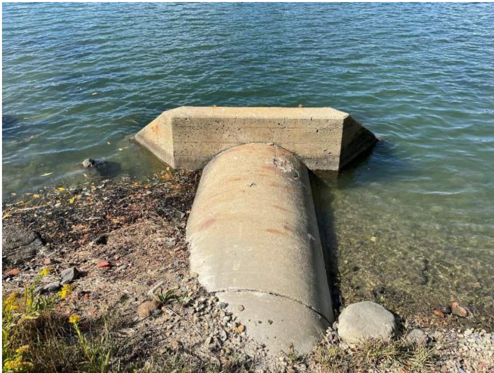
Photo 2 – Existing outfall headwall and exposed 48” RCP pipe looking northwest at approximate high tide. Taken 9/28/22
