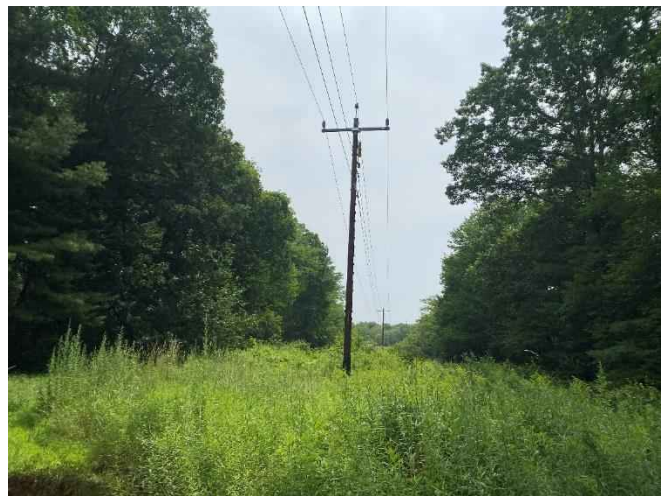
Existing wooden Structure 6 on 339 Distribution Line replaced in 2022.
