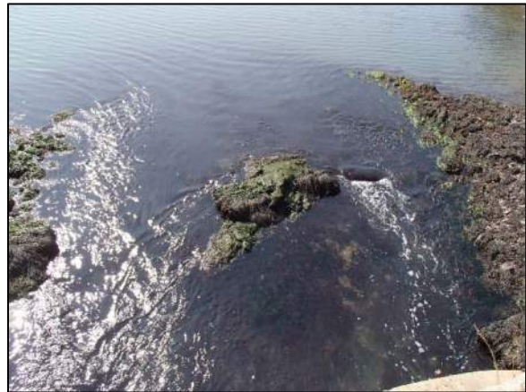
Figure 18 – View south from Maplewood Avenue at the grade control feature just upstream from the bridge inlet (09-23-20)
